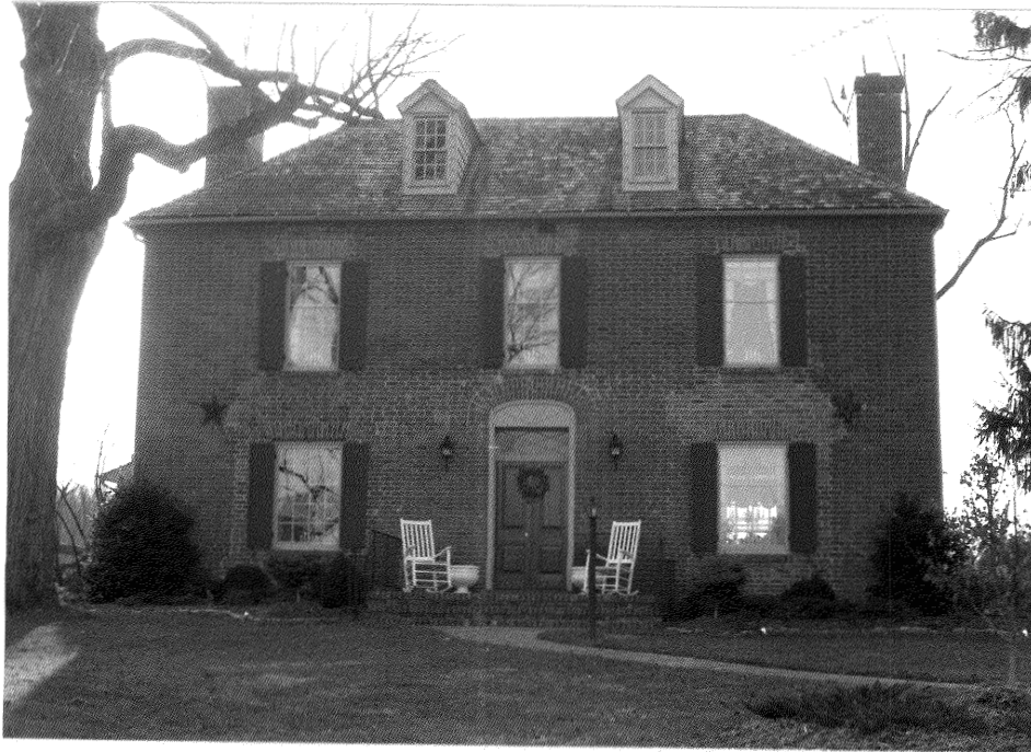
Figure 15: Photograph of Hartwood (89-68), (Traceries, 1992)
