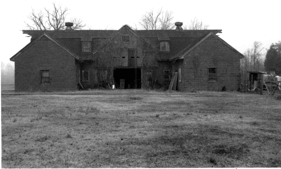
Figure 44: Photograph of Hay Barn/Dairy Barn at Farm on Shackley Point (89-154) (Traceris, 1992)
