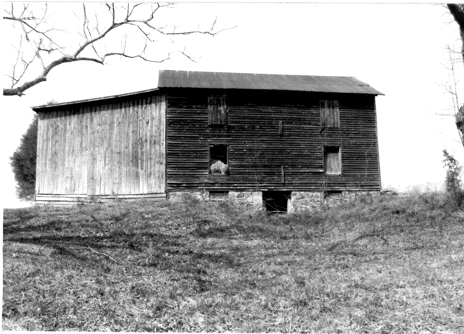
Figure 47: Photograph of Bank Barn at Farm, Route 616 (89-217), (Traceris, 1992)
