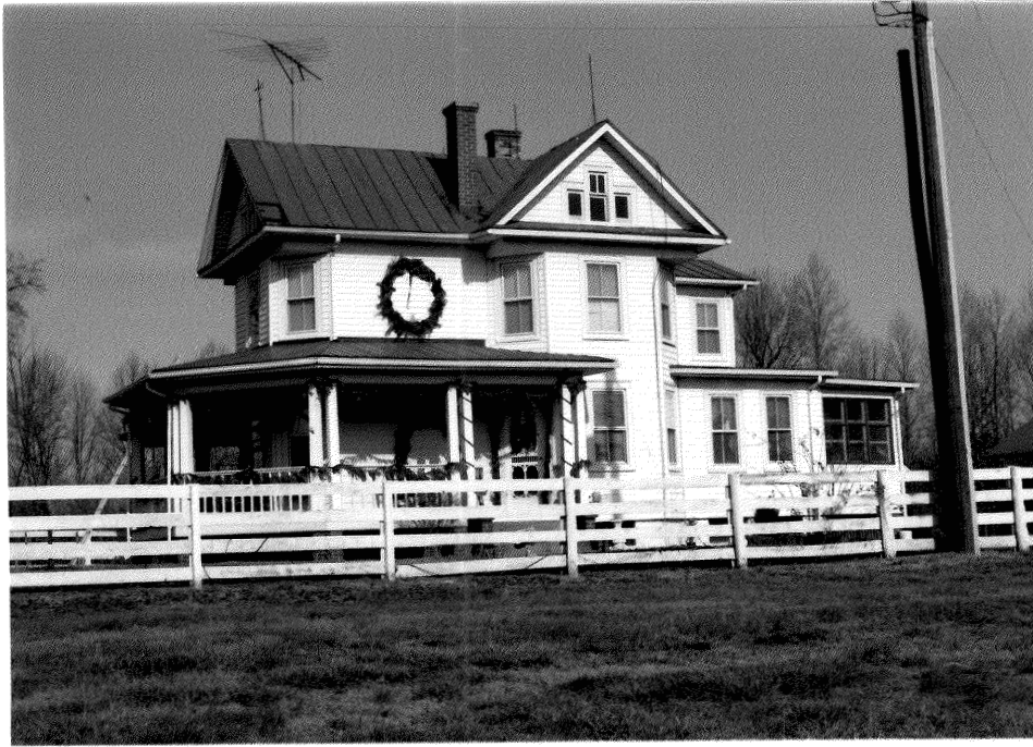
Figure 22: Photograph of House, Hartwood Road (89-127), (Tracerics, 1992)
