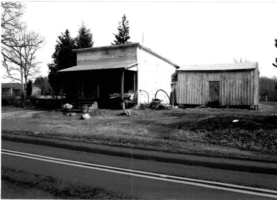
Figure 52: Photograph of Miller Store and Post Office (89-188), (Traceries, 1992)
