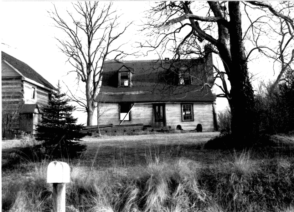
Figure 7: Photograph of Concord (89-97), (Traceries, 1991)
